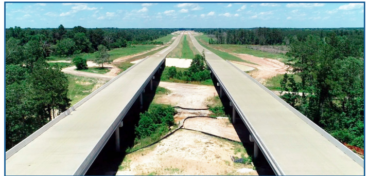
8-mile-long I-69 Diboll Relief Route south of Lufkin to be completed in the fall of 2025.
